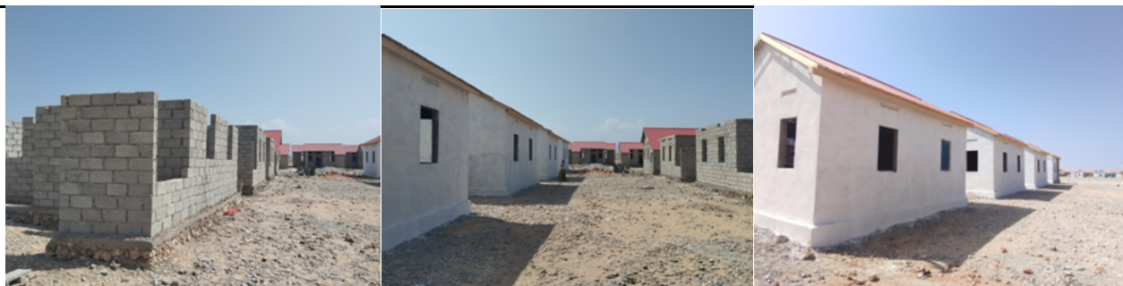
Figure 7: Newly constructed housing units in Gribble, Bosaso
