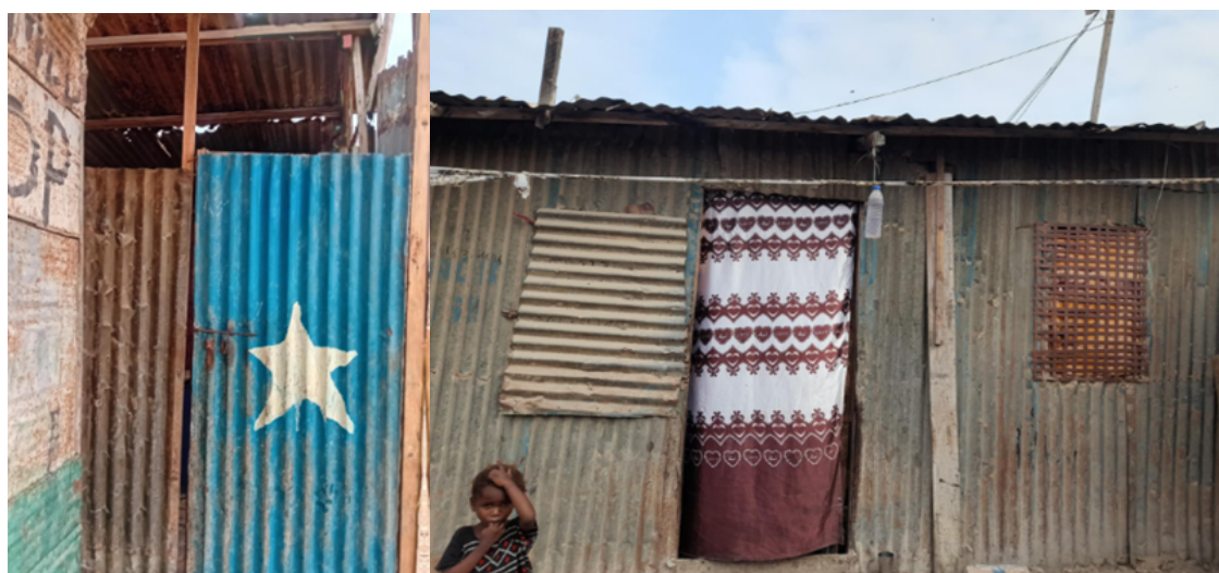
Figure 2: Exterior condition of surveyed Households (UN-Habitat, 2025)
